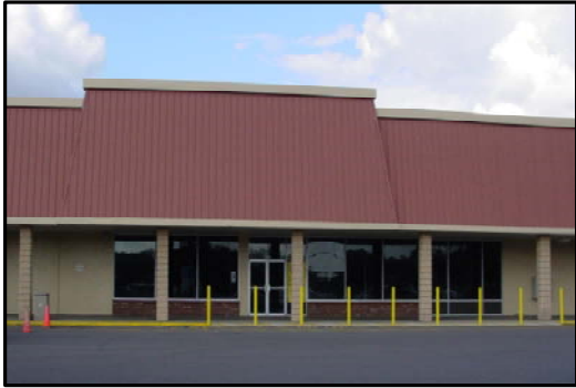
(four) 7.5 ton ac units
